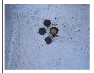
Roof core shows evidence of three course BUR on plywood deck, with indication of dried asphalt.
